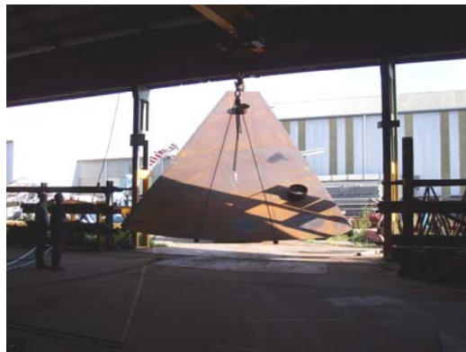
Kellyville roof being positioned
