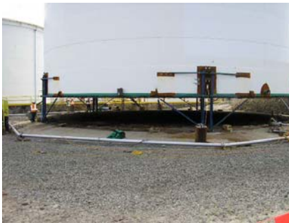
Above & Below Tank Jacking – BP, Perth
