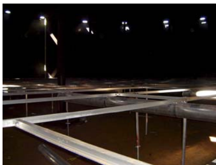
Installation of Aluminium Floating Covers
