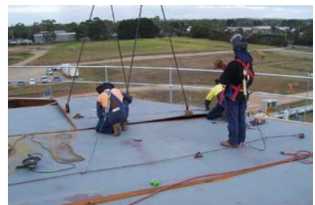
Placing Roof Plates – Hastings, VIC
