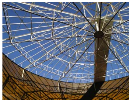
Commencing Roof Plating on Self Supporting Truss Roof Caltex, Gladstone
