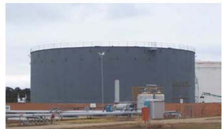
41.4m dia x 14.4m high Cone Roof API Tank with Aluminium Internal Floating Roof Hastings, VIC
