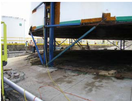
Above & Below Tank Jacking – BP, Perth
