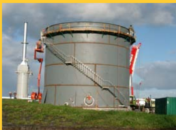
Construction of a Condensate Tank R4 - Lang Lang, VIC
