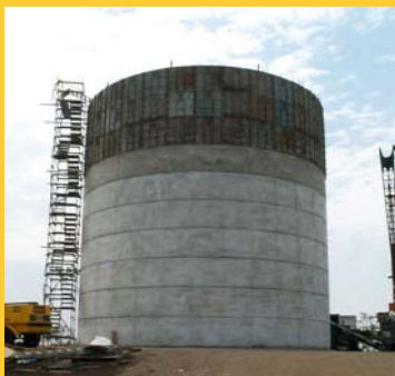
Construction of a 1.4ML Concrete Reservoir Capella, QLD
